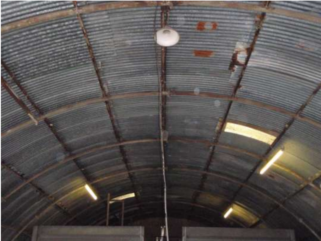
Plate 5. View of roof
