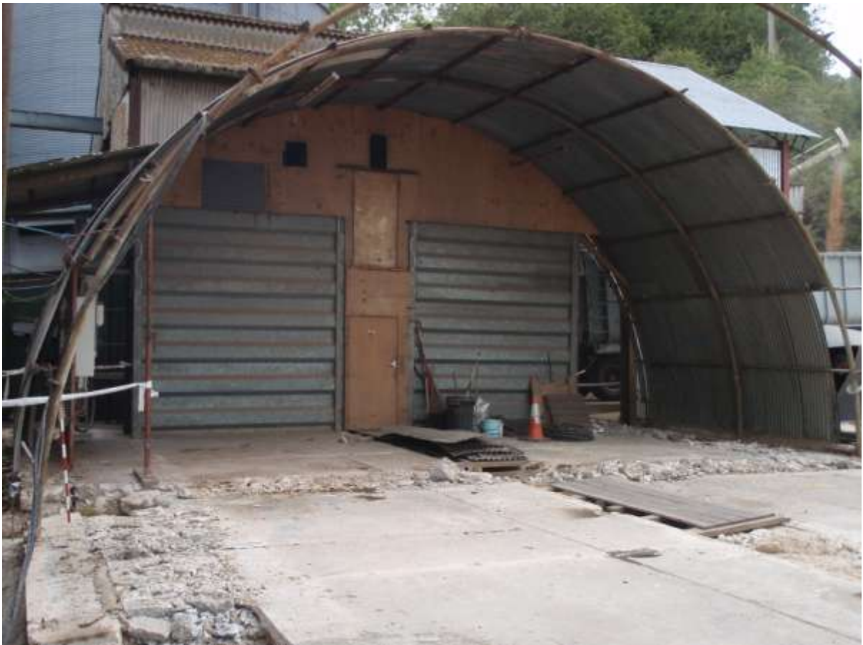
Plate 4. Rear view of building (NNE)
