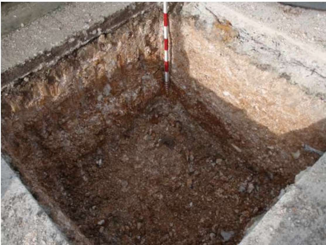
Plate 7. View of the ground reduction post pads (looking NW)
