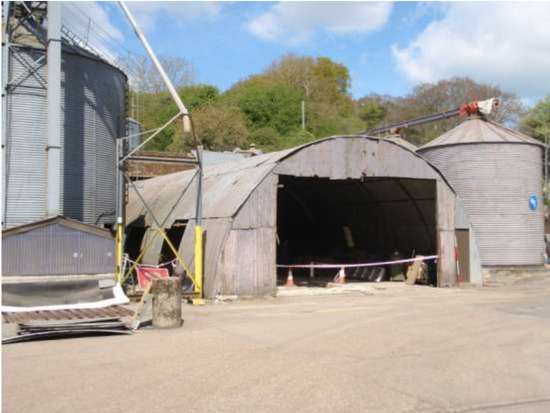
Plate 2. Side view of front elevation (looking NNE)
