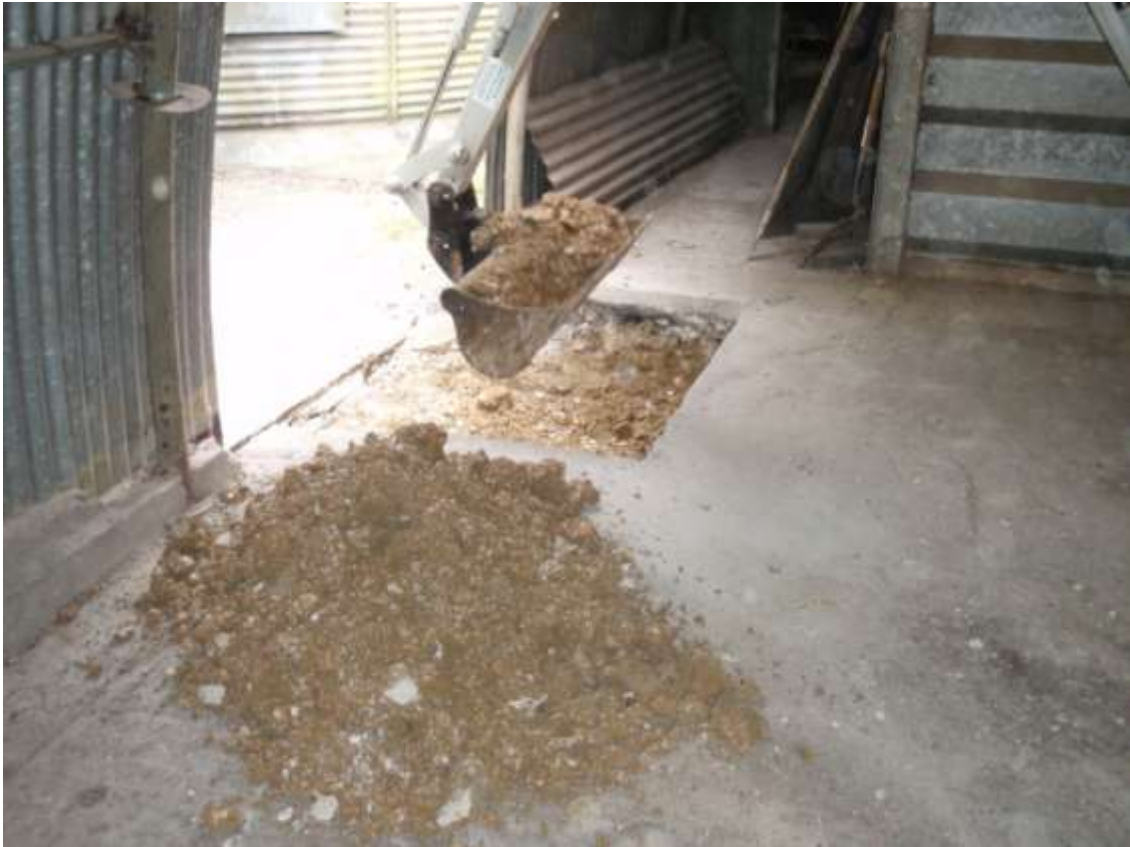
Plate 4. View of ground excavation for concrete pads (looking SW)
