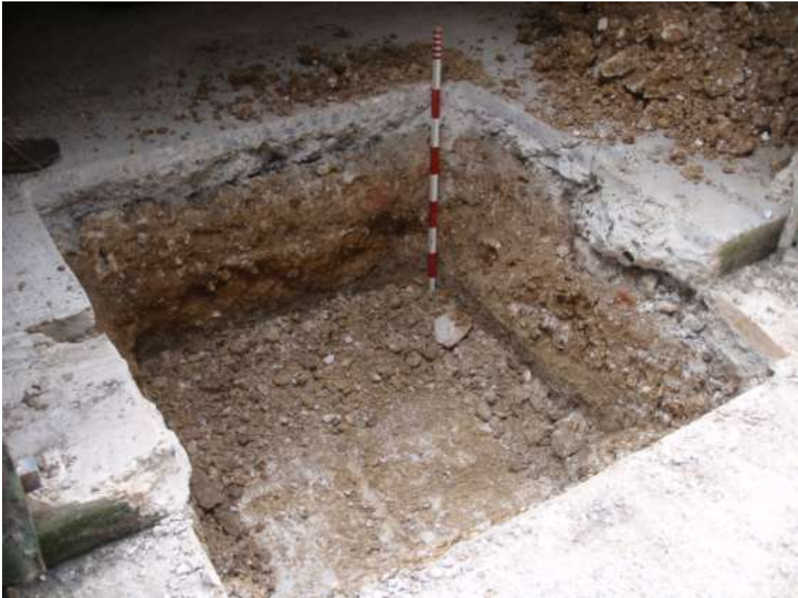
Plate 8. View of the ground reduction post pads (looking NW)
