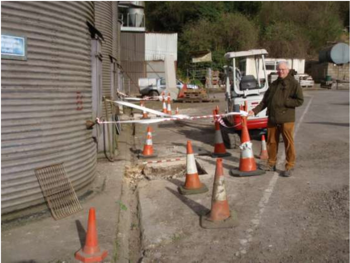
Plate 5. View of post pad excavation (looking NW)
