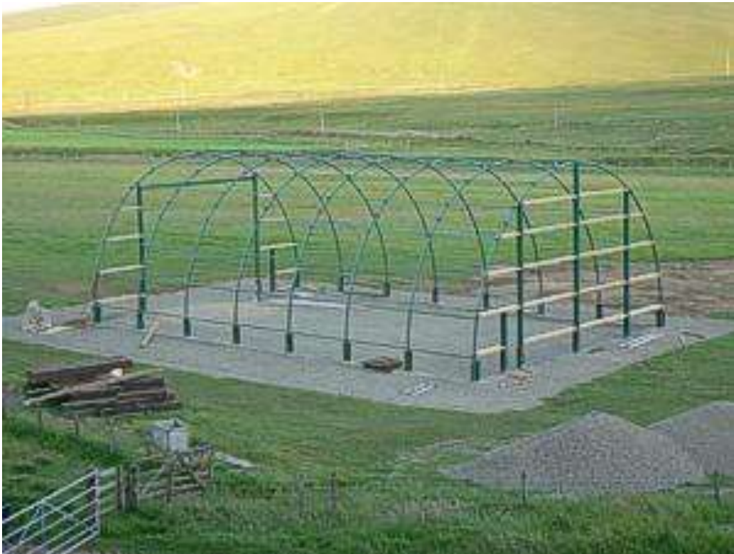
Archive photograph of typical build sequence
