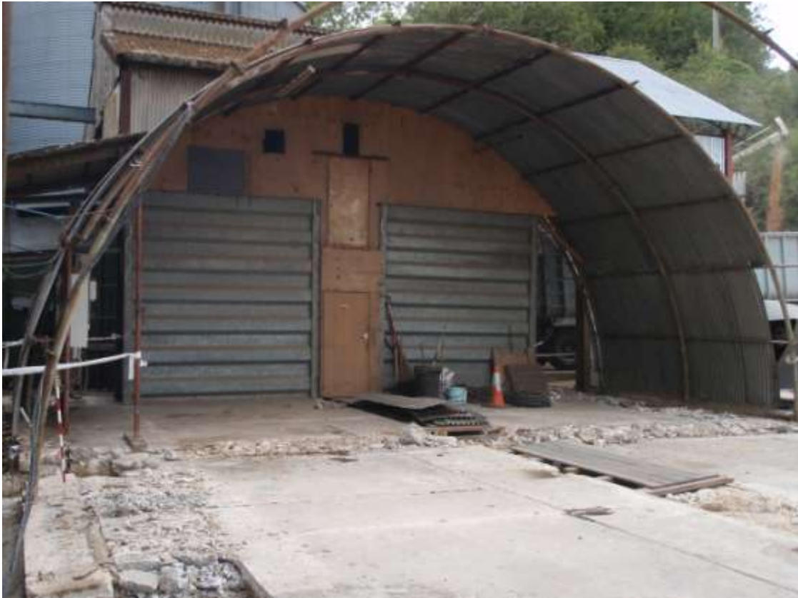
Plate 2. View of site (looking N)
